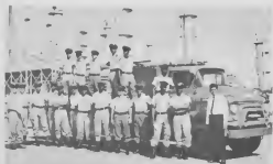
Policemen recently touring refinery pose here with one of Lago's ten firetrucks.
